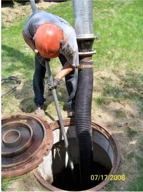
A maintenance worker stationed on the surface uses a vacuum hose to evacuate water, sediment, and floatables from the Jellyfish Filter by inserting the vacuum wand through the maintenance access wall opening.
