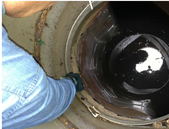
A view of a Jellyfish Filter cartridge deck from the surface showing all the cartridge lids intact and no standing water on the deck (left image), and inspection of the flexible separator skirt from inside the maintenance access wall opening (right image).
