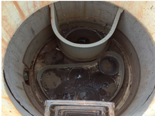
A view of a Jellyfish Filter cartridge deck from the surface showing all the cartridge lids intact and no standing water on the deck (left image), and inspection of the flexible separator skirt from inside the maintenance access wall opening (right image).
